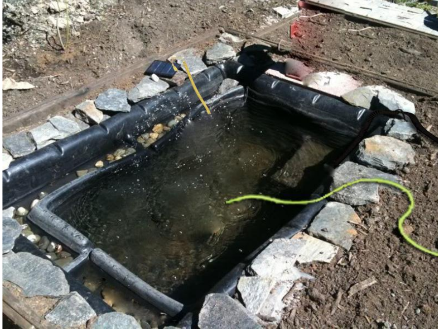
Fig. 3. Construction of experimental salt-gradient solar pond
